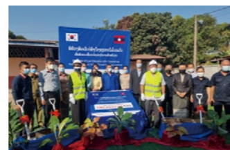
Construction of elementary school in Laos
